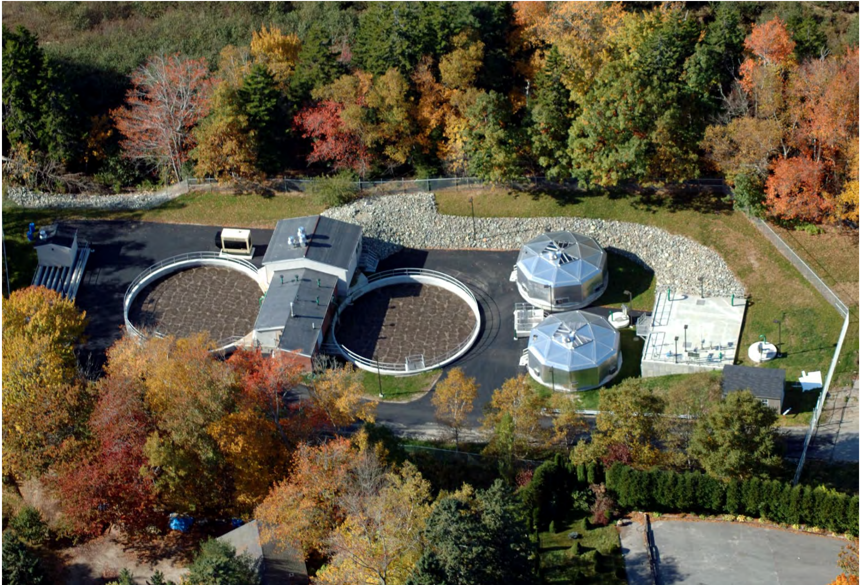
SEAL HARBOR WASTEWATER TREATMENT PLANT
