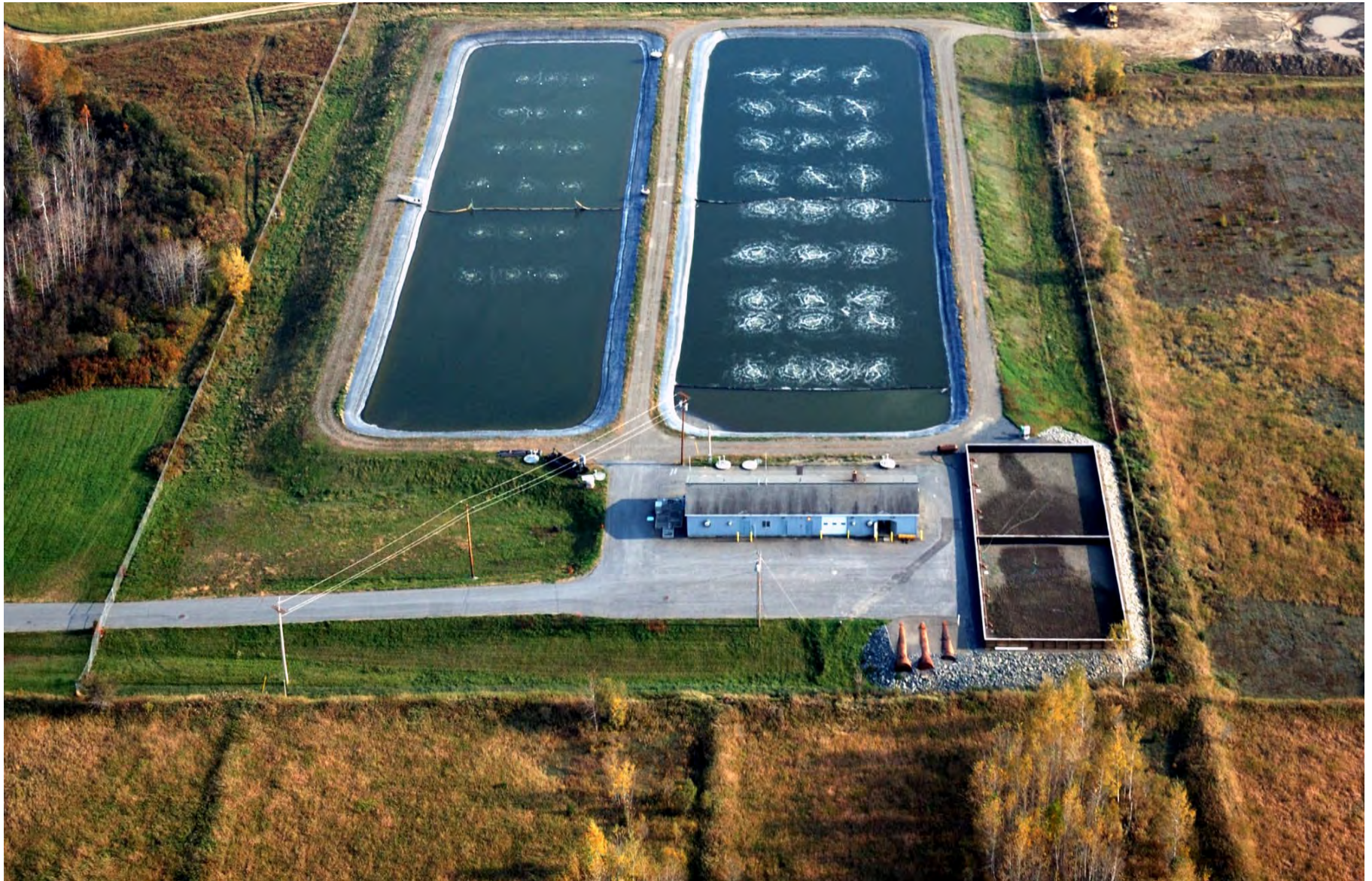
WASHBURN WASTEWATER TREATMENT PLANT
