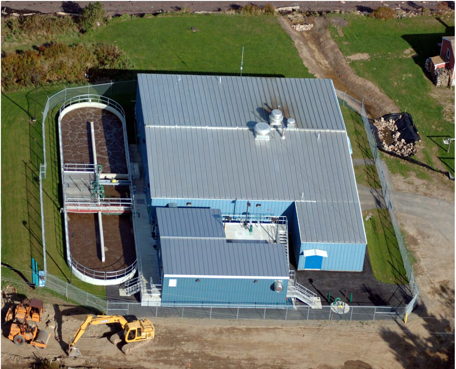
PLEASANT POINT WASTEWATER TREATMENT PLANT
