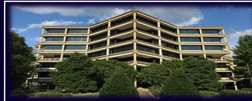
Reston National Center
