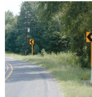
Chevron signs with retroreflective strips on sign posts installed along a curve. Source: FHWA
