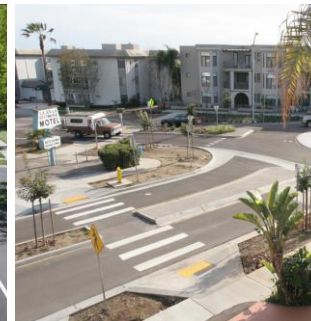
Median and pedestrian refuge island near a roundabout. Source: www.pedbikemages.org / Dan Burden
