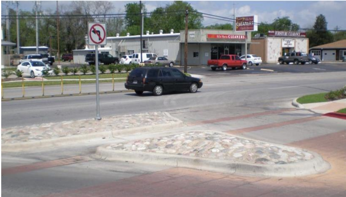
Driveway curbing with “no left turn” sign
